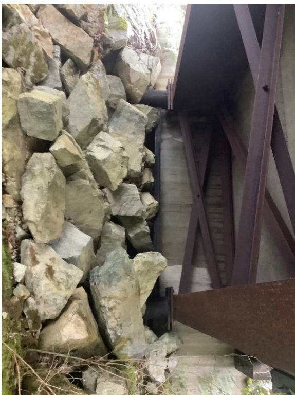
Right Bank Abutment when facing downstream
